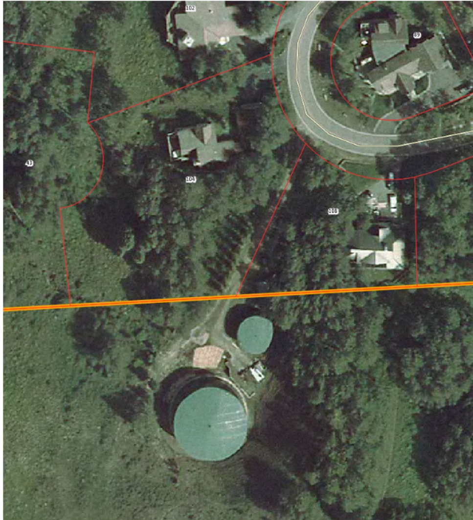
Figure 1. Aerial view of the Timberland Tanks 1 & 2 Sites.
