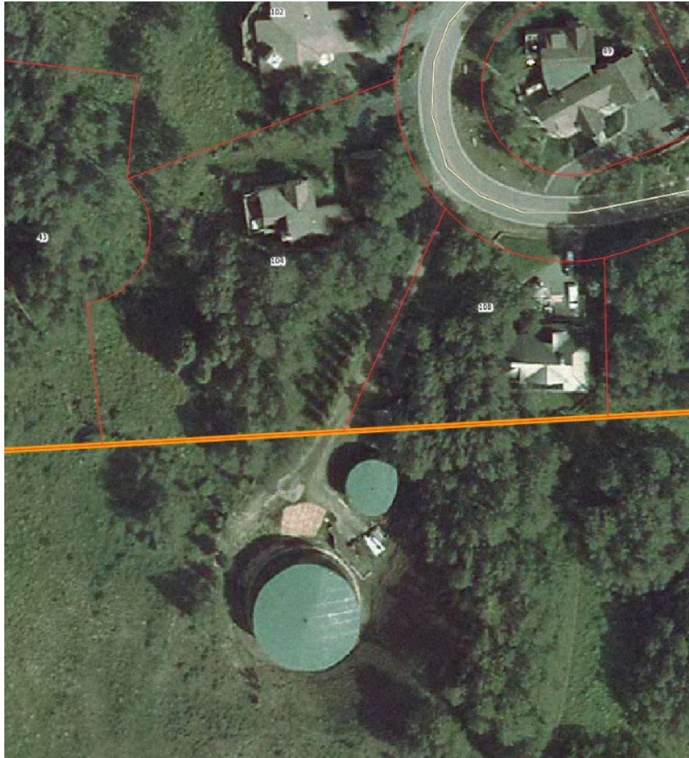
Figure 1. Aerial view of the Timberland Tanks 1 & 2 Sites.
