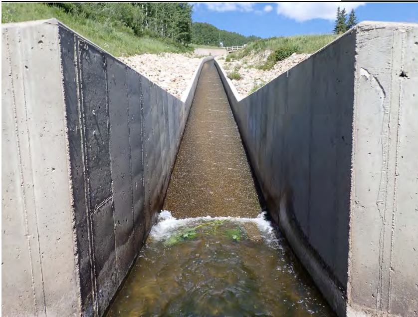
View looking upstream in lower portion of emergency spillway low-flow channel.
