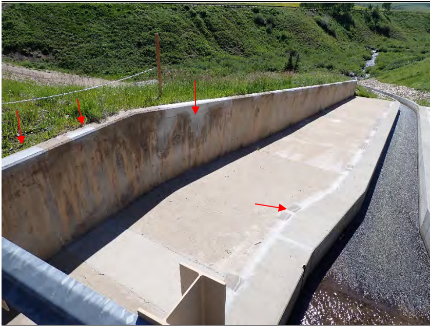
View looking down from bridge crossing at emergency spillway shoot.
