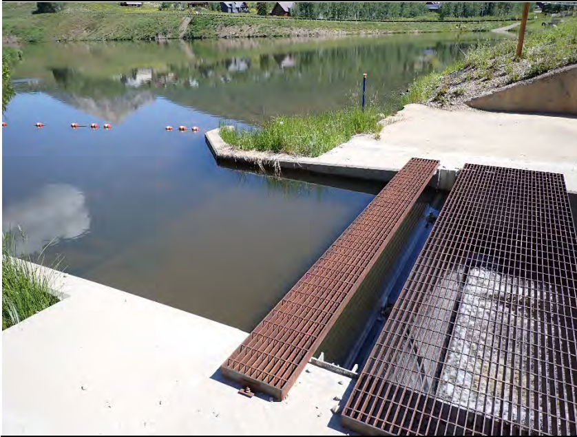
Emergency spillway entrance.
