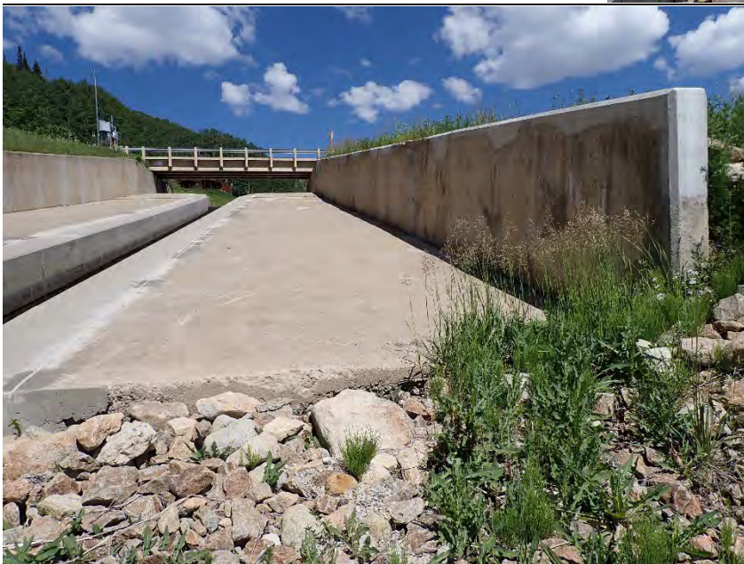
Downstream end of emergency spillway chute.
