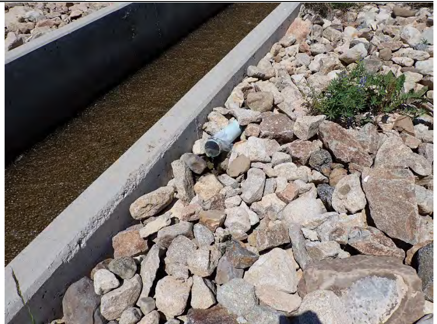
Typical low flow channel transverse joint drain outfall (left side shown).
