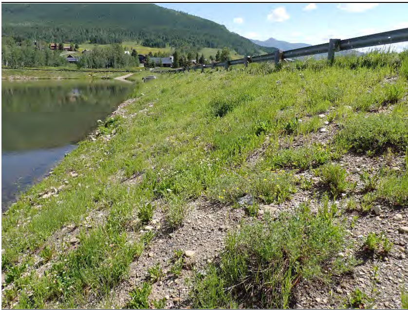
Typical view along upstream slope.
